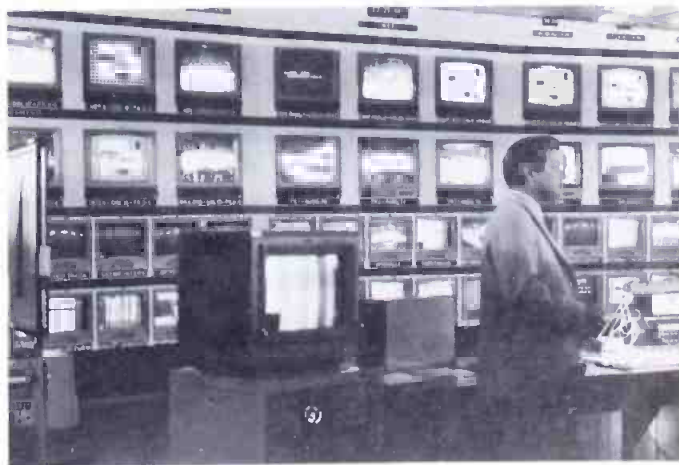
Central switching room at DOZ center provided constant checking on inputs from venues. Labeled by venue along venue along the bottom two rows and by destination on the top two rows.
