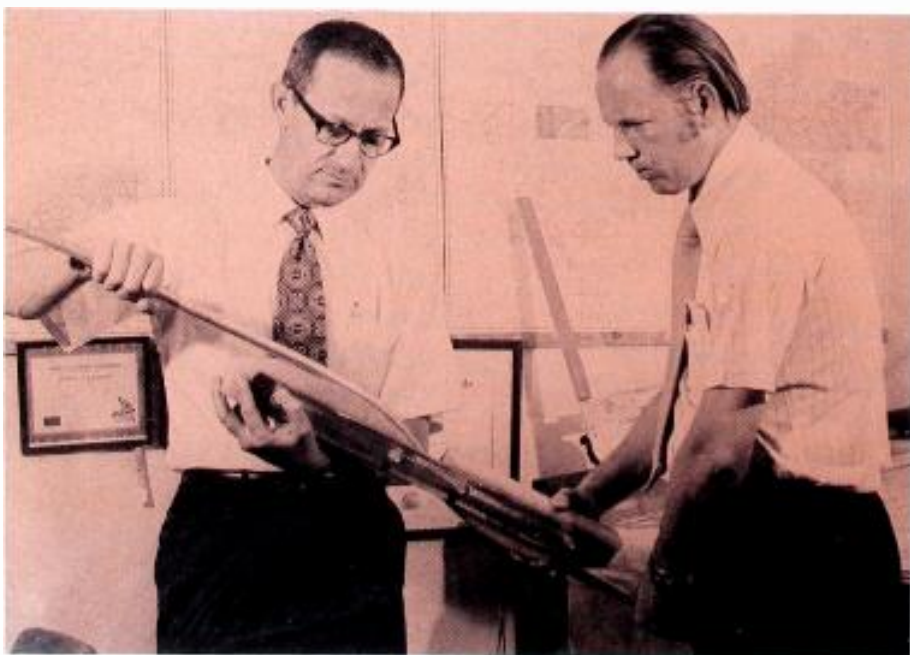
Fig. 1 Electronic systems manager Jim Wright (L) and Don Ellis inspect a \frac{3}{4} -inch cable bender for use at Cable TV of Rockford.
